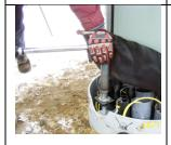
4. Diagonally, proceed in tightening, starting with the last nuts installed in step 2, WITH A TORQUE WRENCH adjusted to 120 ft-lb. Once completed, insert a (half) jam nut on top of each of the tightened nuts and tighten the jam nuts slightly by hand with an open wrench. IMPORTANT: DO NOT torque the jam nuts with a the torque wrench.
