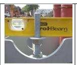
1. If applicable, take off the (red) safety cover and then the plastic sleeves on the four threaded rods protruding from the Sub-base. Insert a nut then a flat washer (supplied in a bag in one of the upper compartments of the cabinet) onto each of the four threaded rods. Position the nuts so that each of the flat washers is at the level of the top of the Sub-base (see photo).
