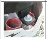
3. Insert a flat washer and a standard nut on every threaded rod. Diagonally, tighten all nuts by hand with an open wrench (approx. equiv. to 60 ft-lb). Make sure the cabinet has remained perfectly level. If not level, loosen the upper nuts and REPEAT STEP 2 to correct level of cabinet.
